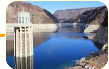
Colorado River Aqueduct
