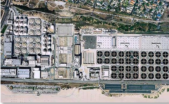
Hyperion Water Reclamation Plant City of Los Angeles
