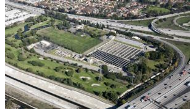
Los Coyotes Water Reclamation Plant Sanitation Districts of LA County
