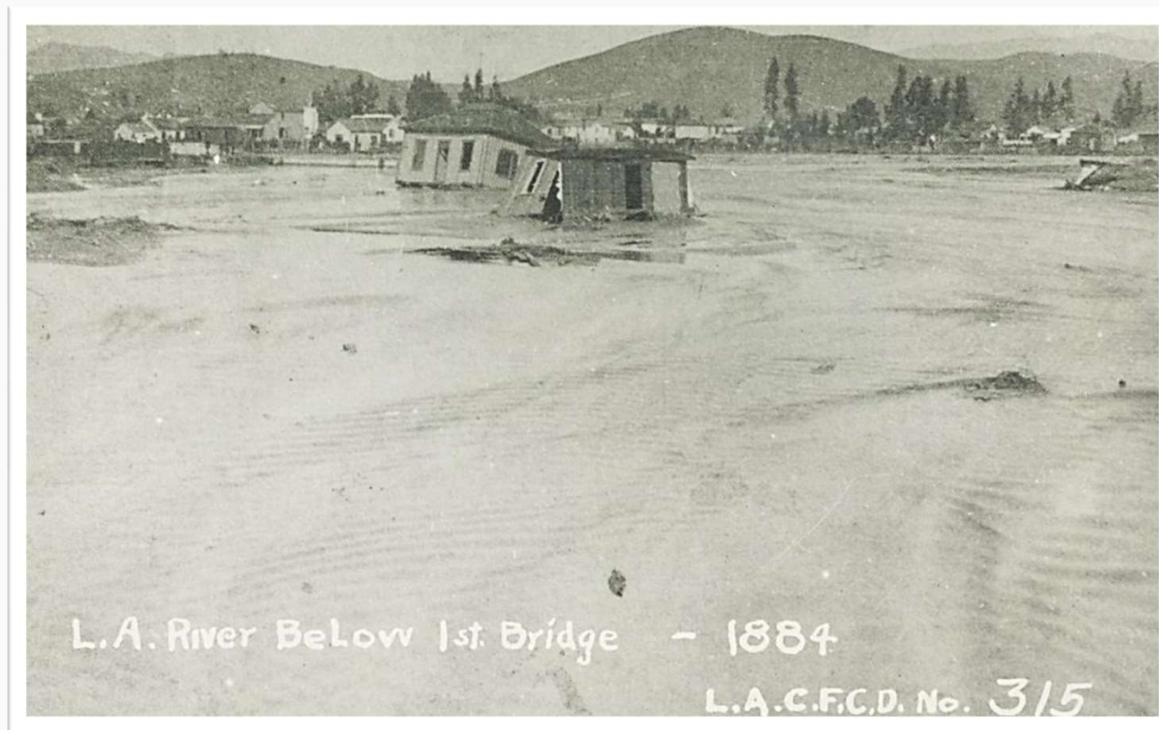
Los Angeles River south of First Street
